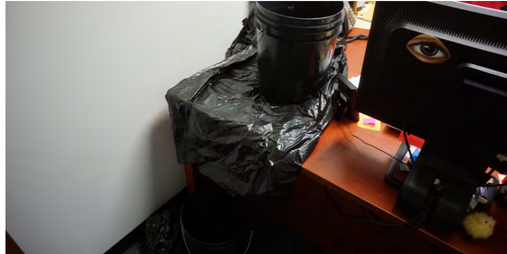
Roof leaks are apparent during storms and other events; staff has taken to using 5-gallon buckets in many of the rooms to help catch water during rainfall.
