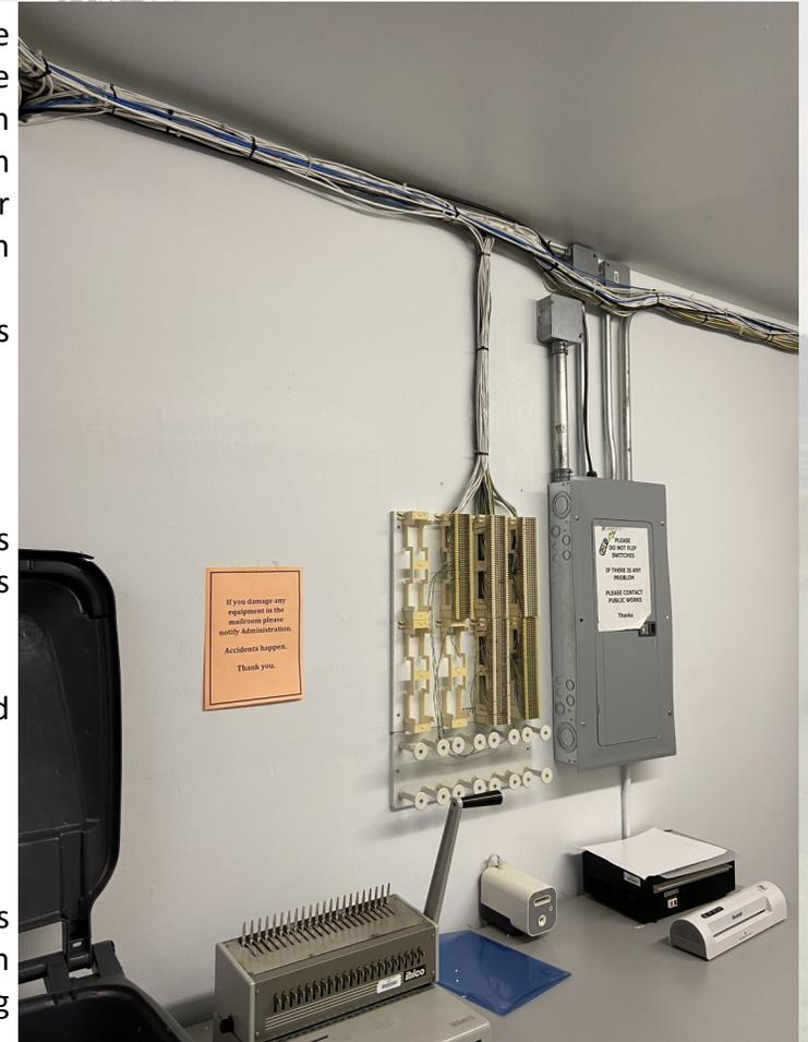
Figure 8-3. Exposed wiring in City Hall
