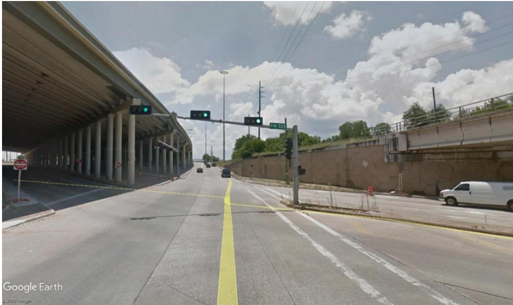
Figure 5. EB US 290 Service Road Approach
