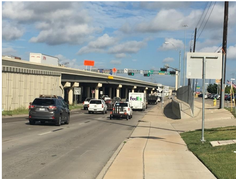
Figure 3. WB US 290 Service Road Approach
