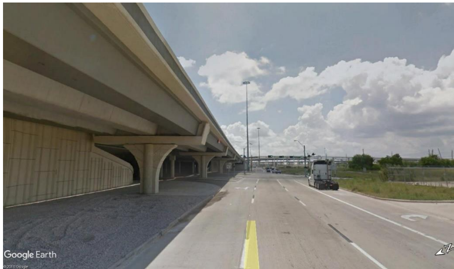
Figure 5. EB US 290 Service Road Approach
