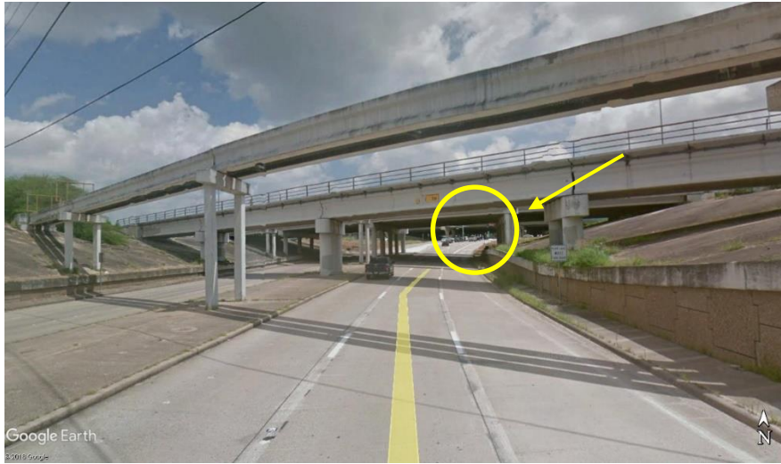
Figure 7. NB Senate Avenue Approach Before Overpass
