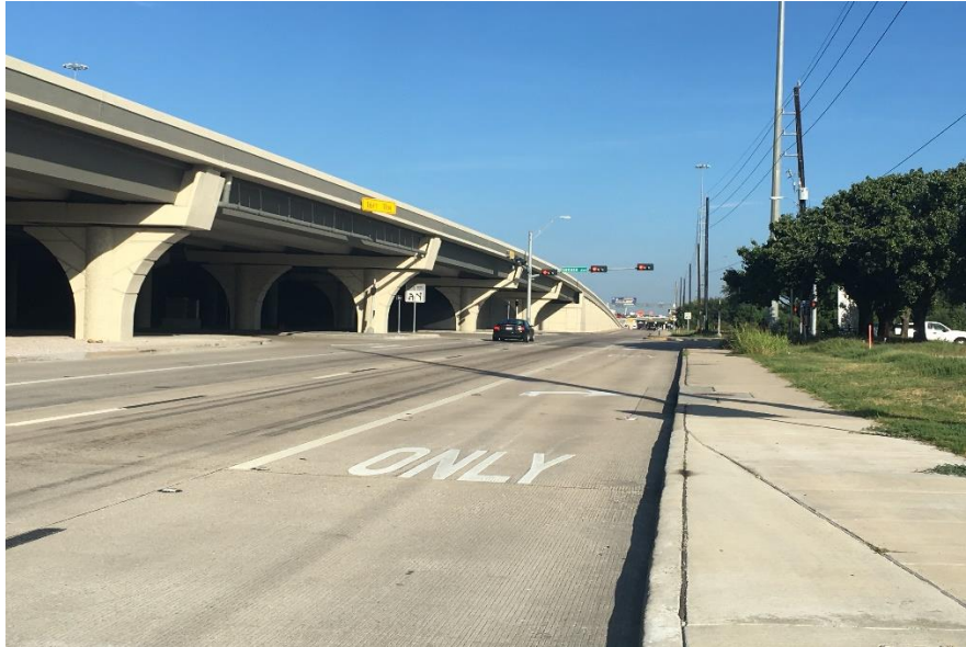
Figure 3. WB US 290 Service Road Approach
