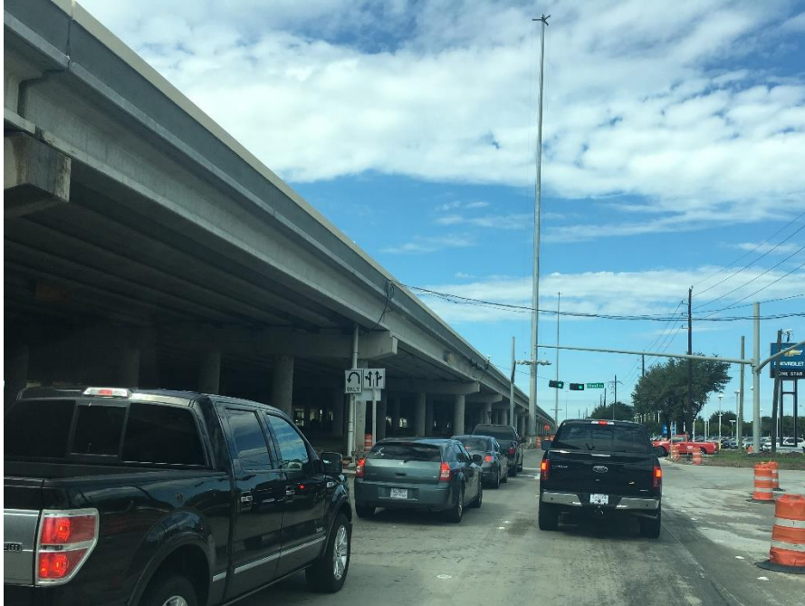
Figure 3. WB US 290 Service Road Approach
