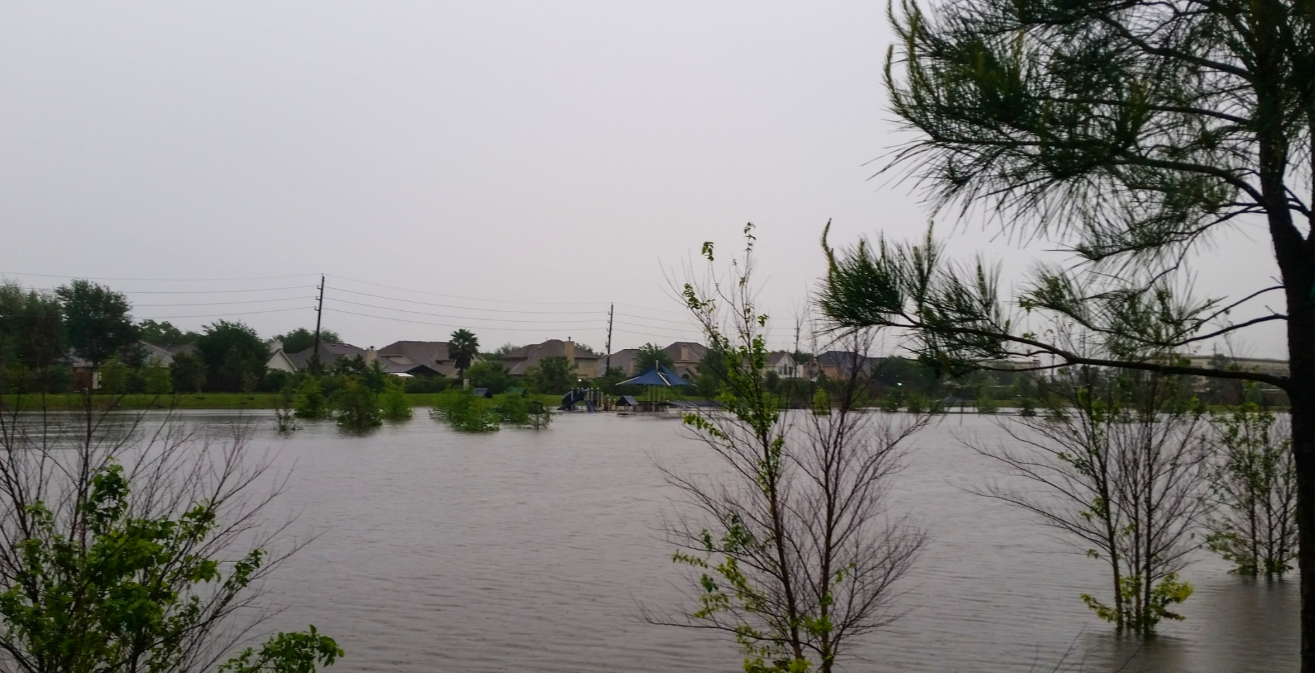
Westwillow Stormwater Detention Basin
