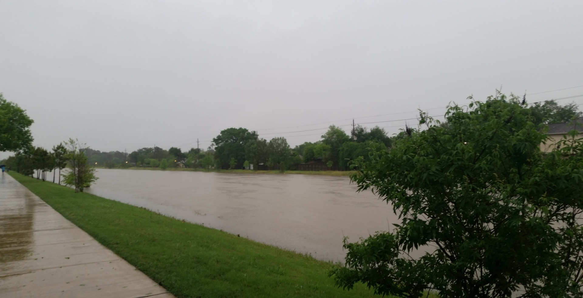
Jersey Village Bypass Channel
